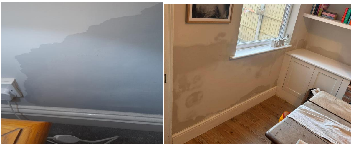
Typical signs of rising dampness with visible tide marks along the walls.
