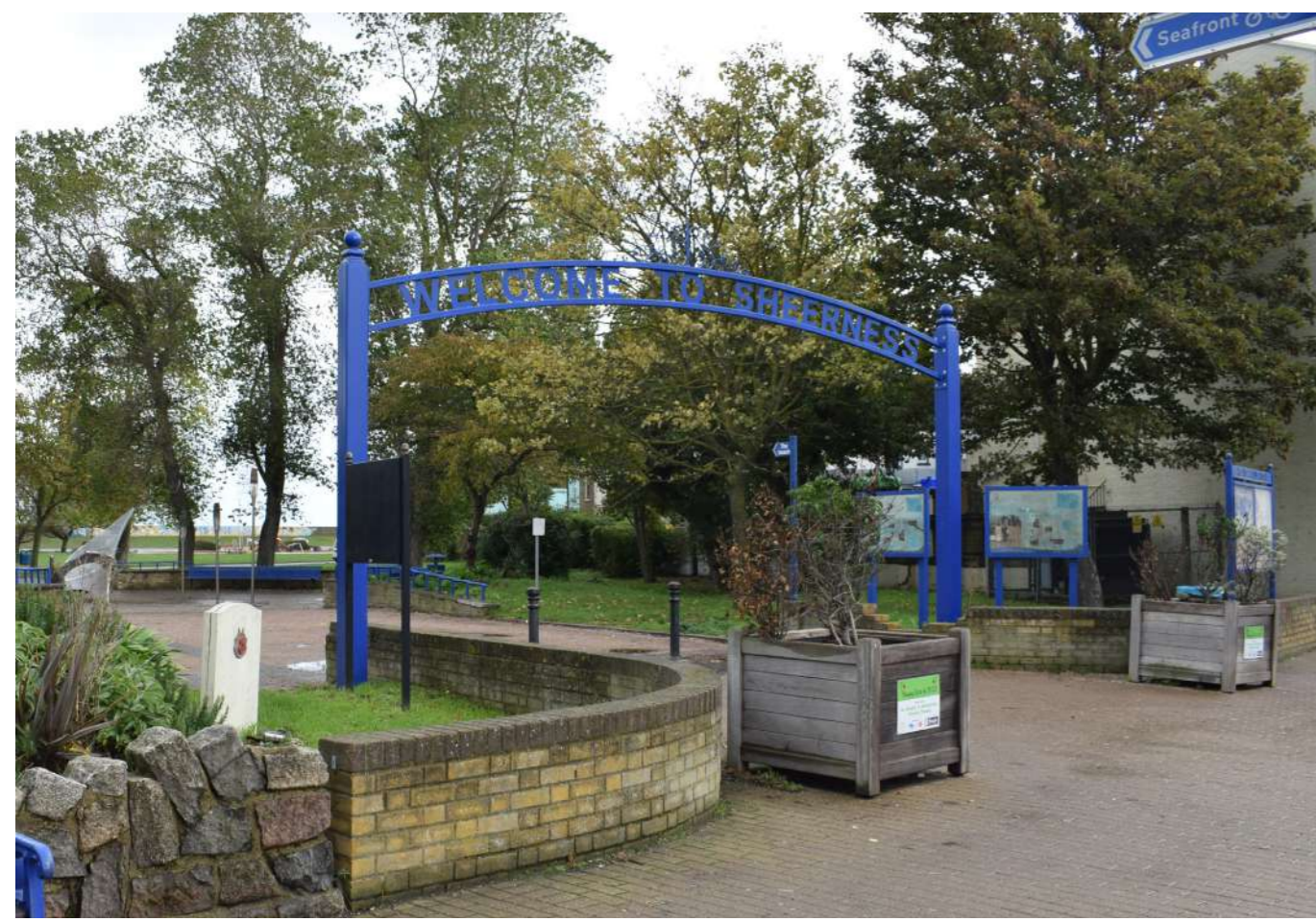
1 Walls pulled back to widen entrance and existing arch to be centred.
